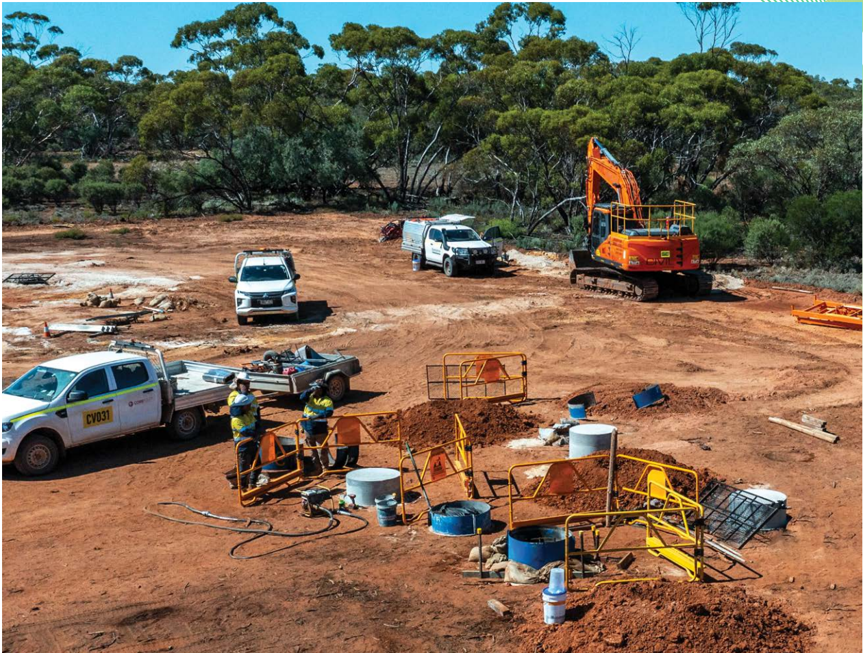
Pictured: Tower foundations being prepared at Project Energy Connect west of Wagga Wagga.
