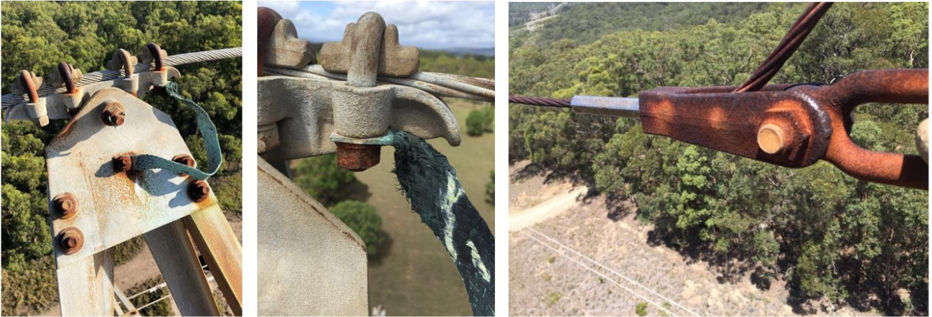
Figure 2-9 Damaged insulators
