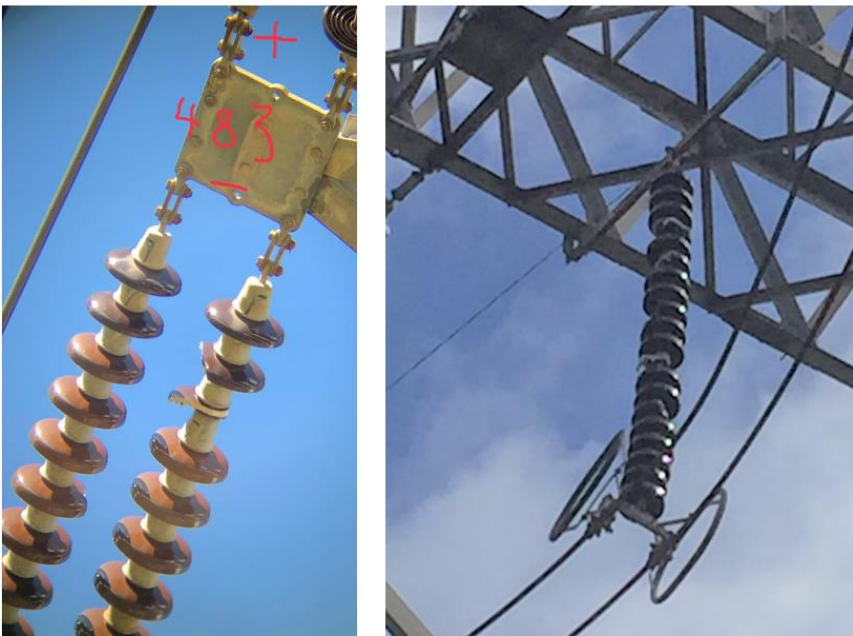
Figure 2-9 Damaged insulators
