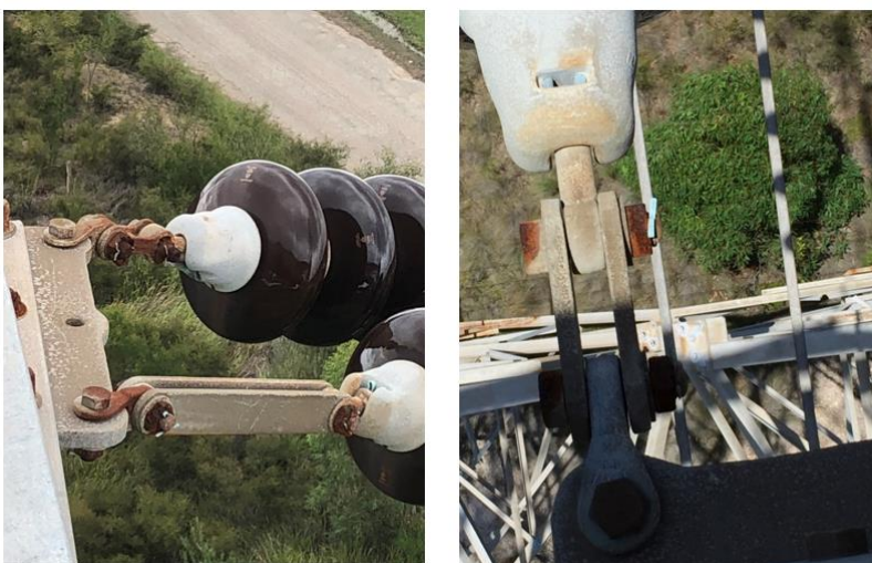
Figure 2-5 Corrosion affecting conductor fitting attachments
