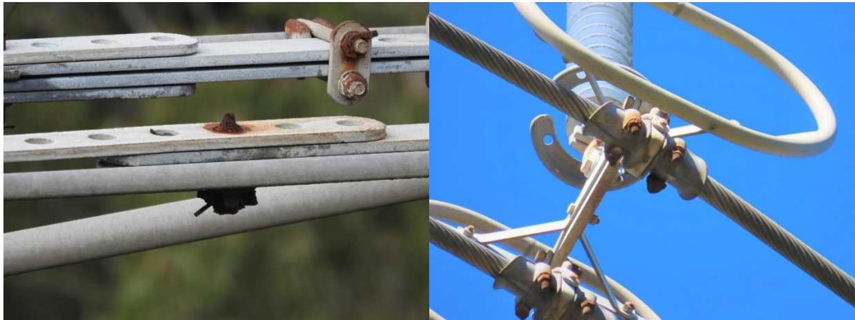
Figure 2.4 Corroded insulator pins
