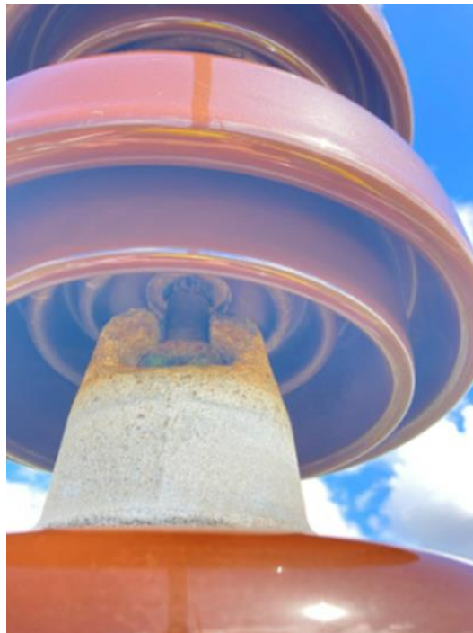
Figure 2.4 Corroded insulator pins
