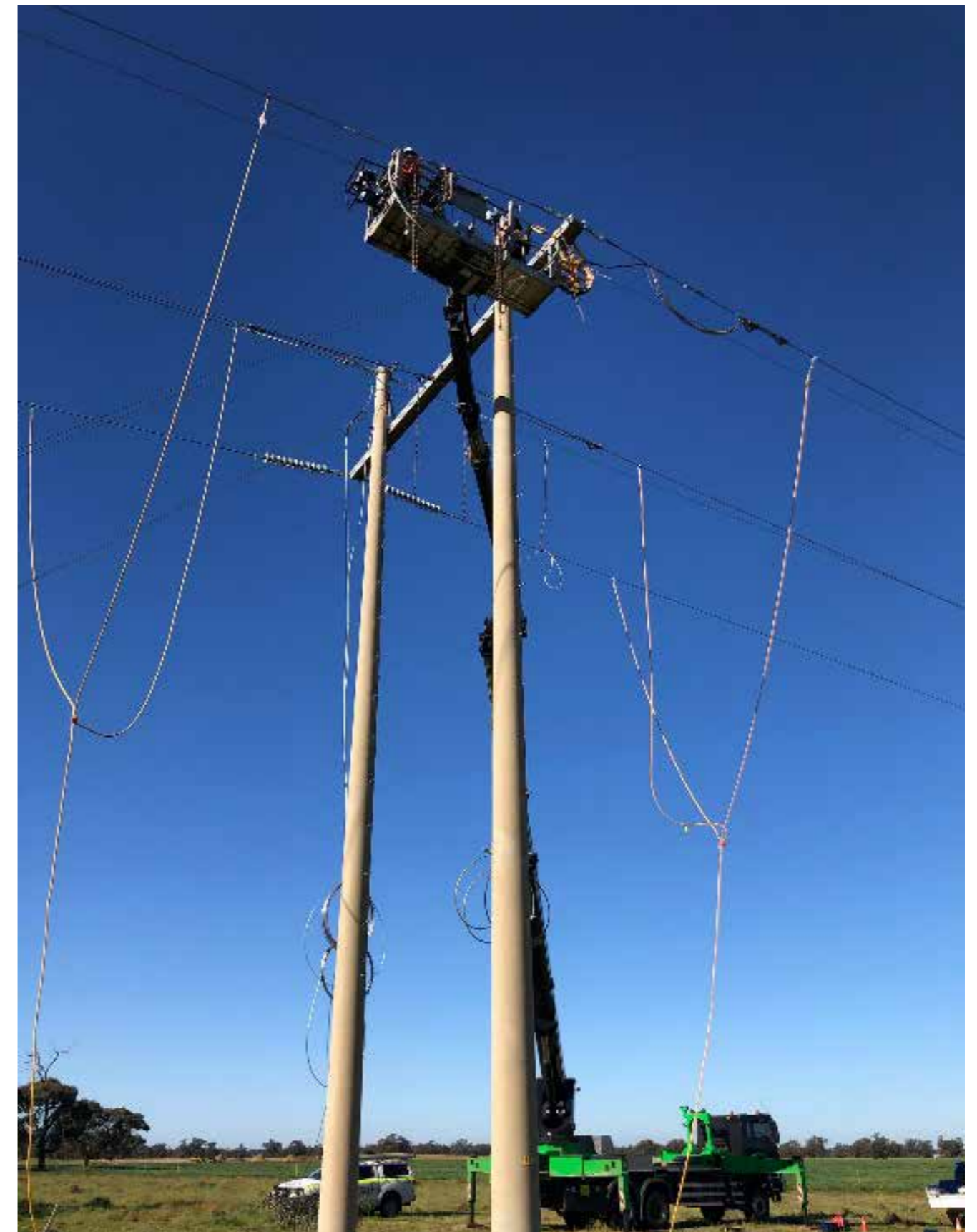
Figure 14-8: Installation of high temperature low sag conductor in Southern NSW
