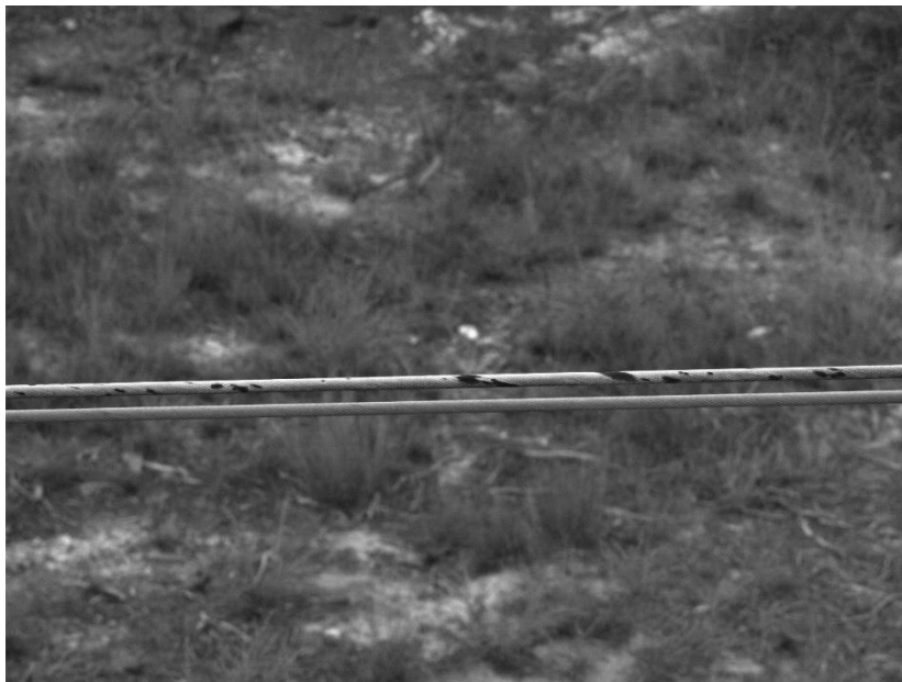
Figure 2-2: Conductor discolouration
