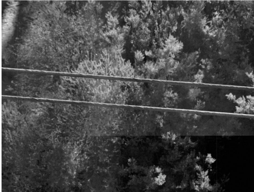
Figure 2-2: Conductor discolouration
