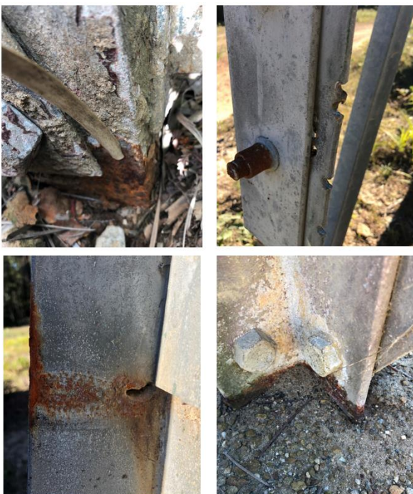
Figure 2-3 Corroded tower members
