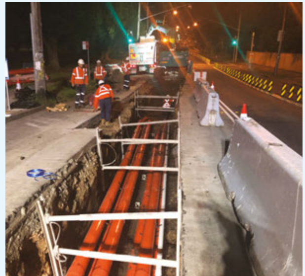
夜间沟槽挖掘施工 (Old Canterbury Road, Ashfield)
