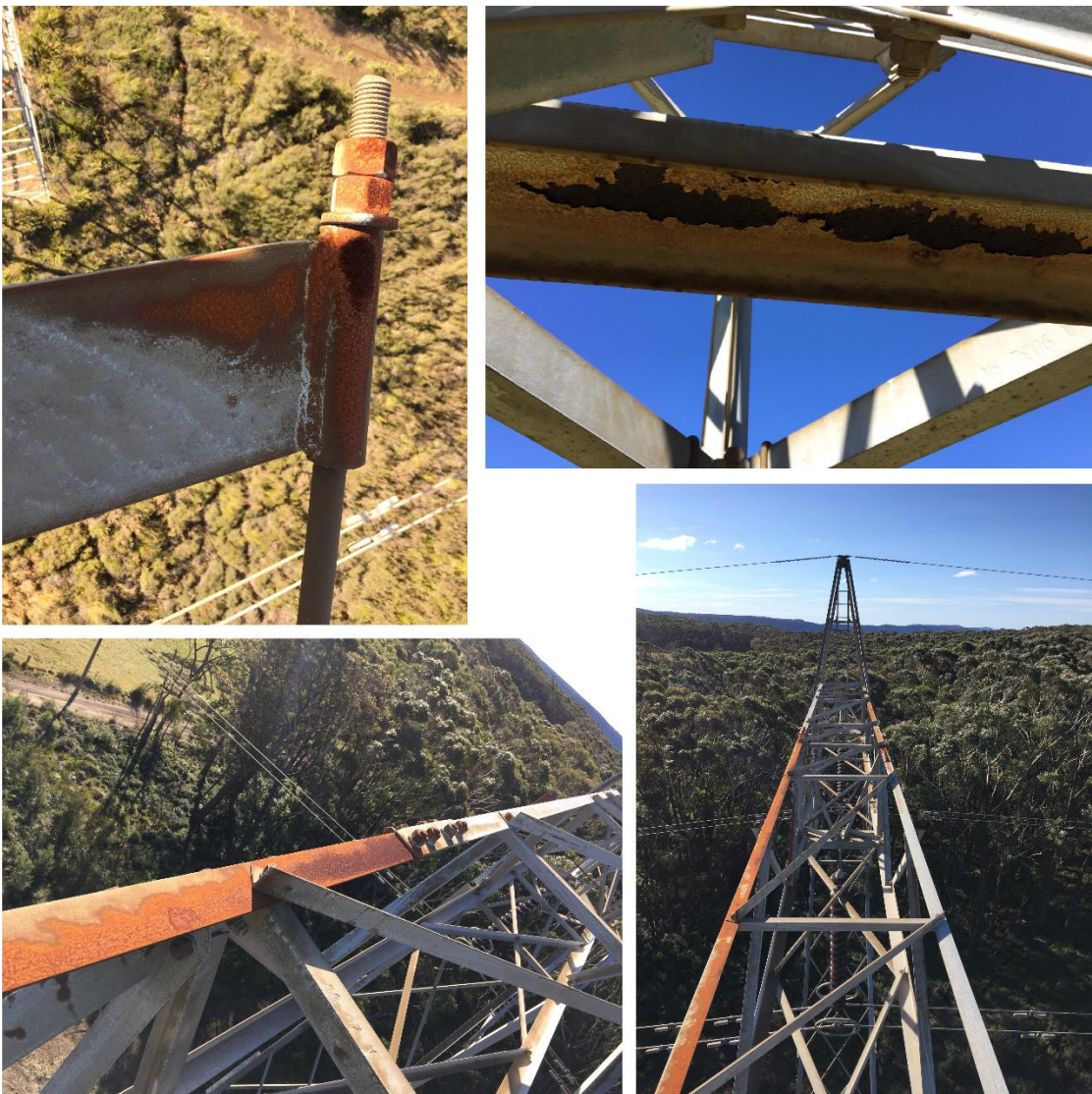
Figure 2-6 Rust on cross-arm members
