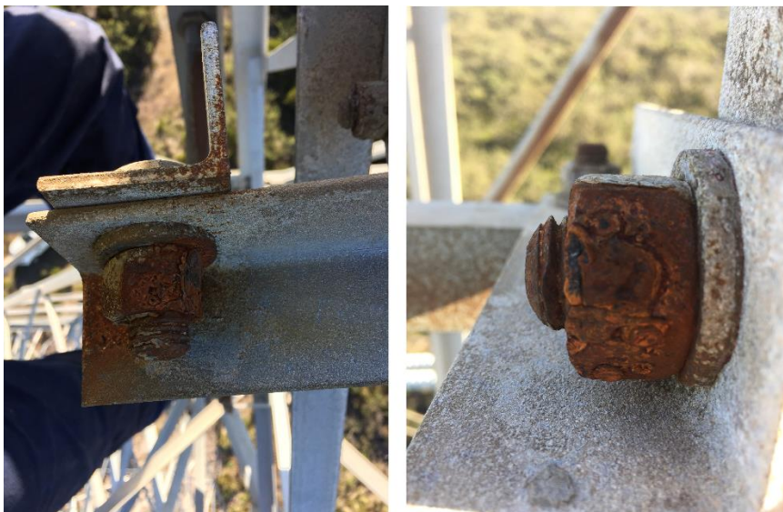
Figure 2-5 Corroded fasteners
