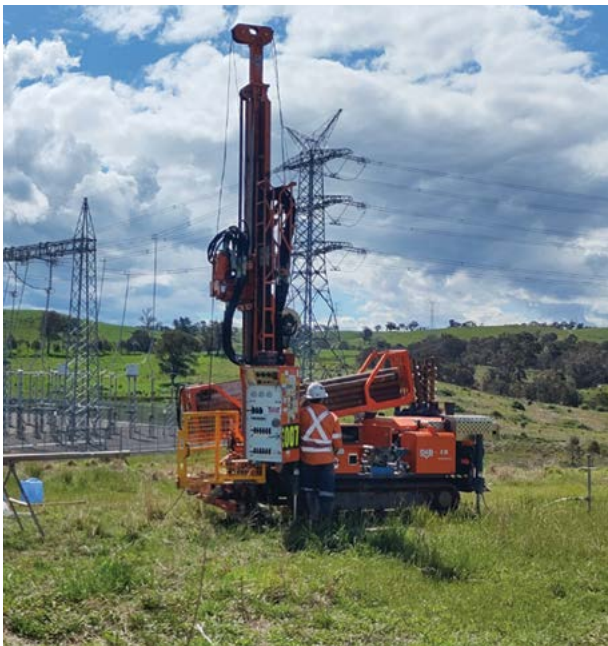
Pictured: Geotechnical investigations at Bannaby substation.
