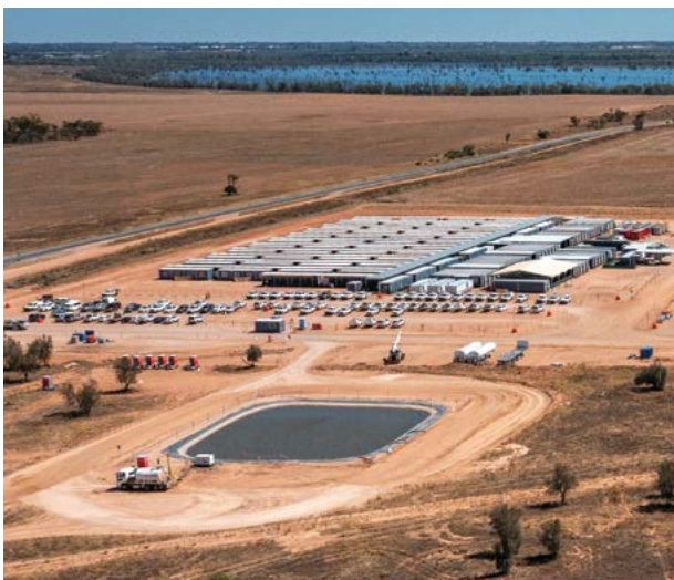
Pictured: Water storage pond located near construction worker accommodation at Project Energy Connect west of Wagga Wagga.
