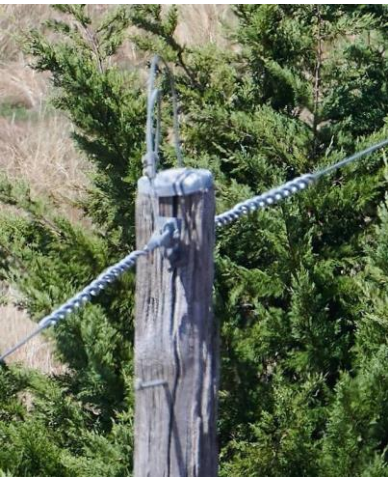
Figure 2-4 Wood pole deterioration
