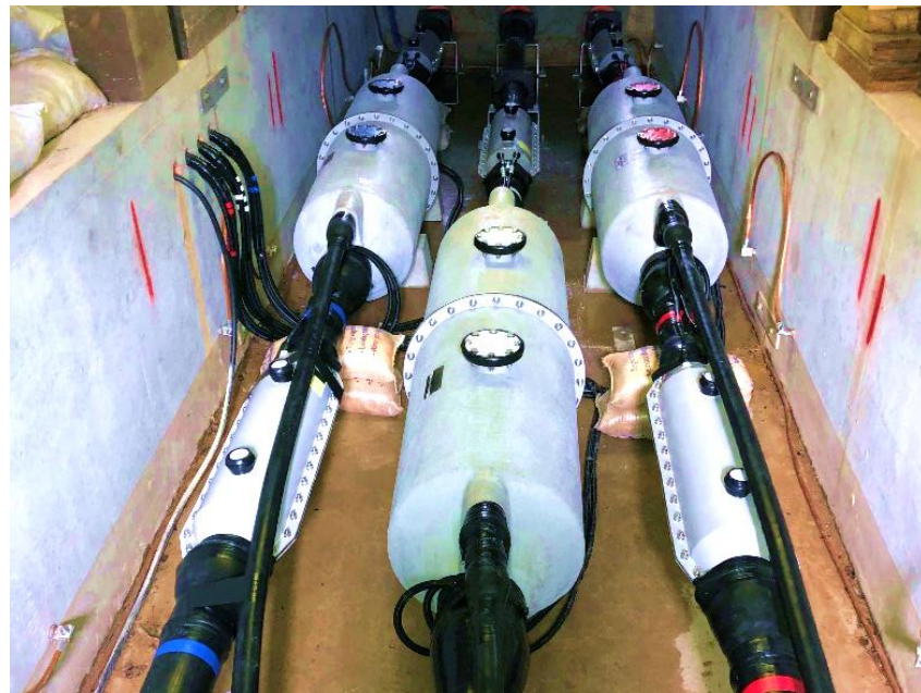
330kV Joints complete at Joint Bay 13/14, Hanks Street Ashfield
