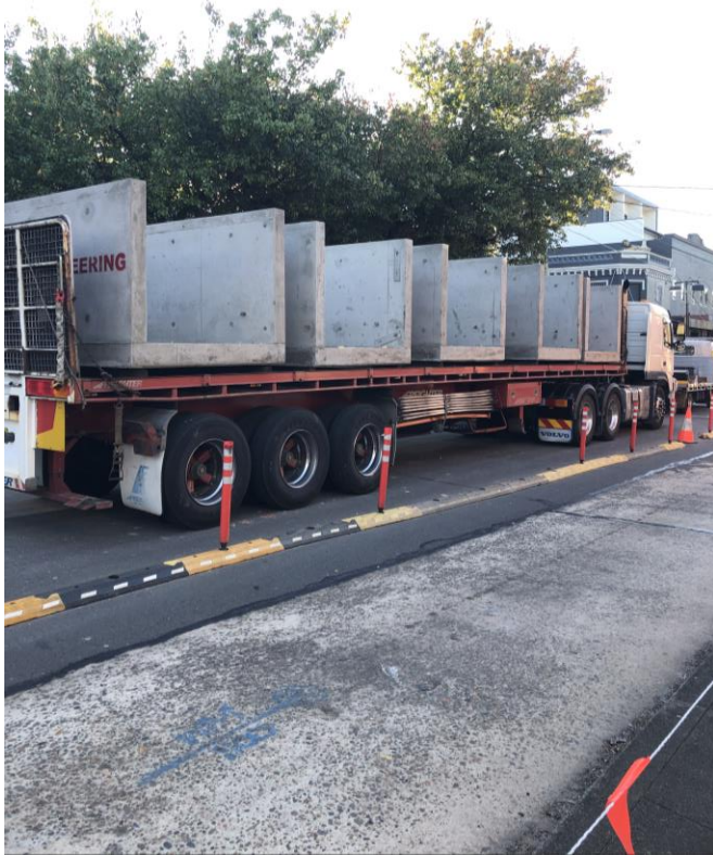
Delivery and installation of joint bay (Cable 47) on Addison Road, Marrickville (April 2021)
