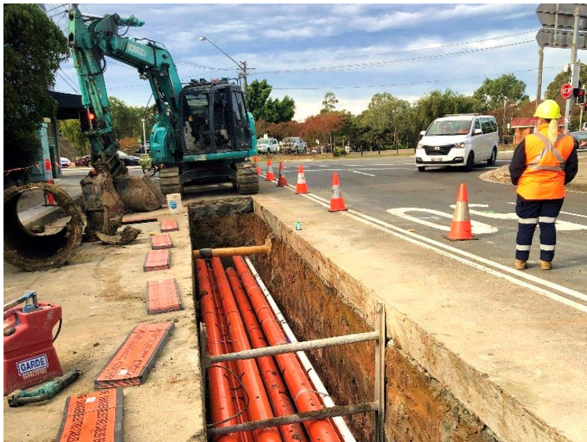
Conduits installed, awaiting backfill – May Street, St Peters
