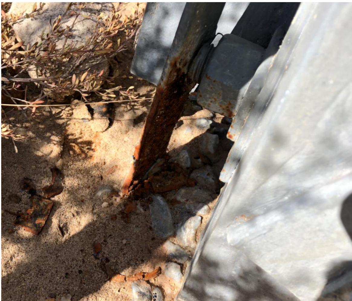
Figure 2-4 Tower earthing issues
