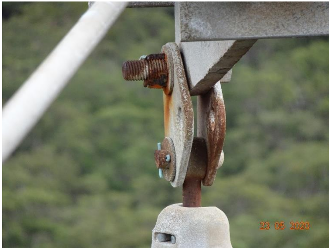
Figure 2-4 Tower earthing issues
