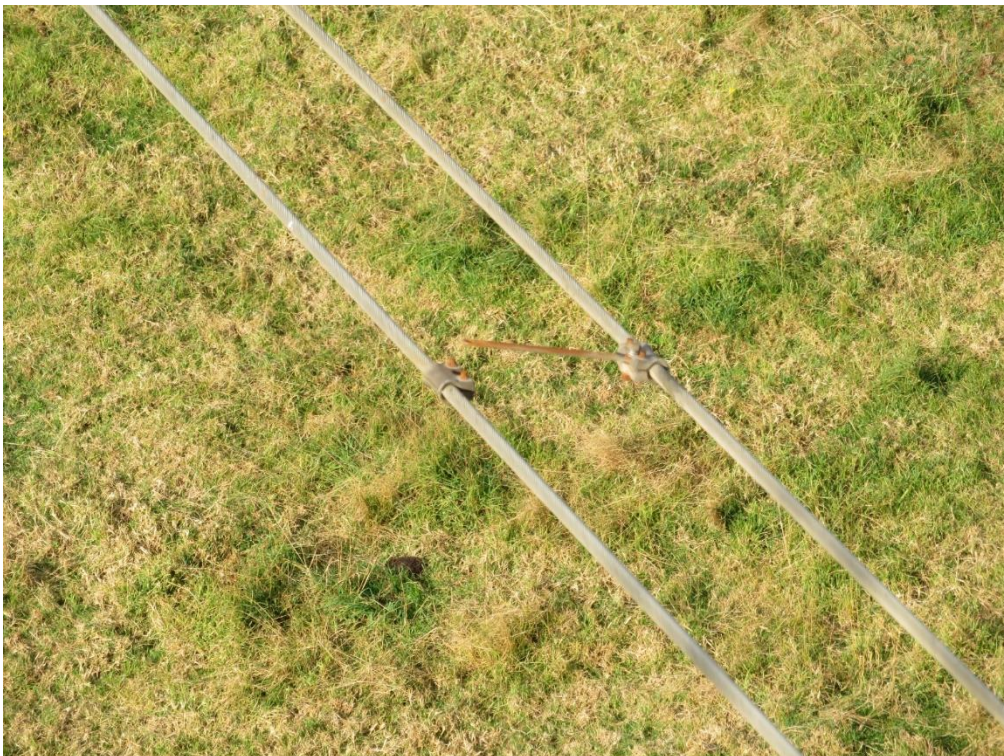
Figure 2-4 Damaged conductor spacers
