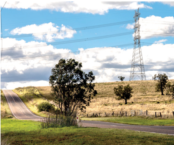
Pictured: 500 kV transmission towers in Muswellbrook.
