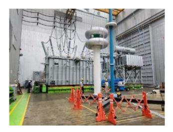
Last year we welcomed the arrival of the 374 tonne Phase Shifting Transformer (PST) for EnergyConnect, the nation-critical project that will unlock greater renewable energy sharing between NSW, South Australia, and Victoria. Not only this is the first 330 kV PST to be installed in Australia, but it is also a specialised transformer that:
