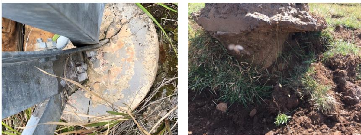
Figure 2-2 Damaged footings
