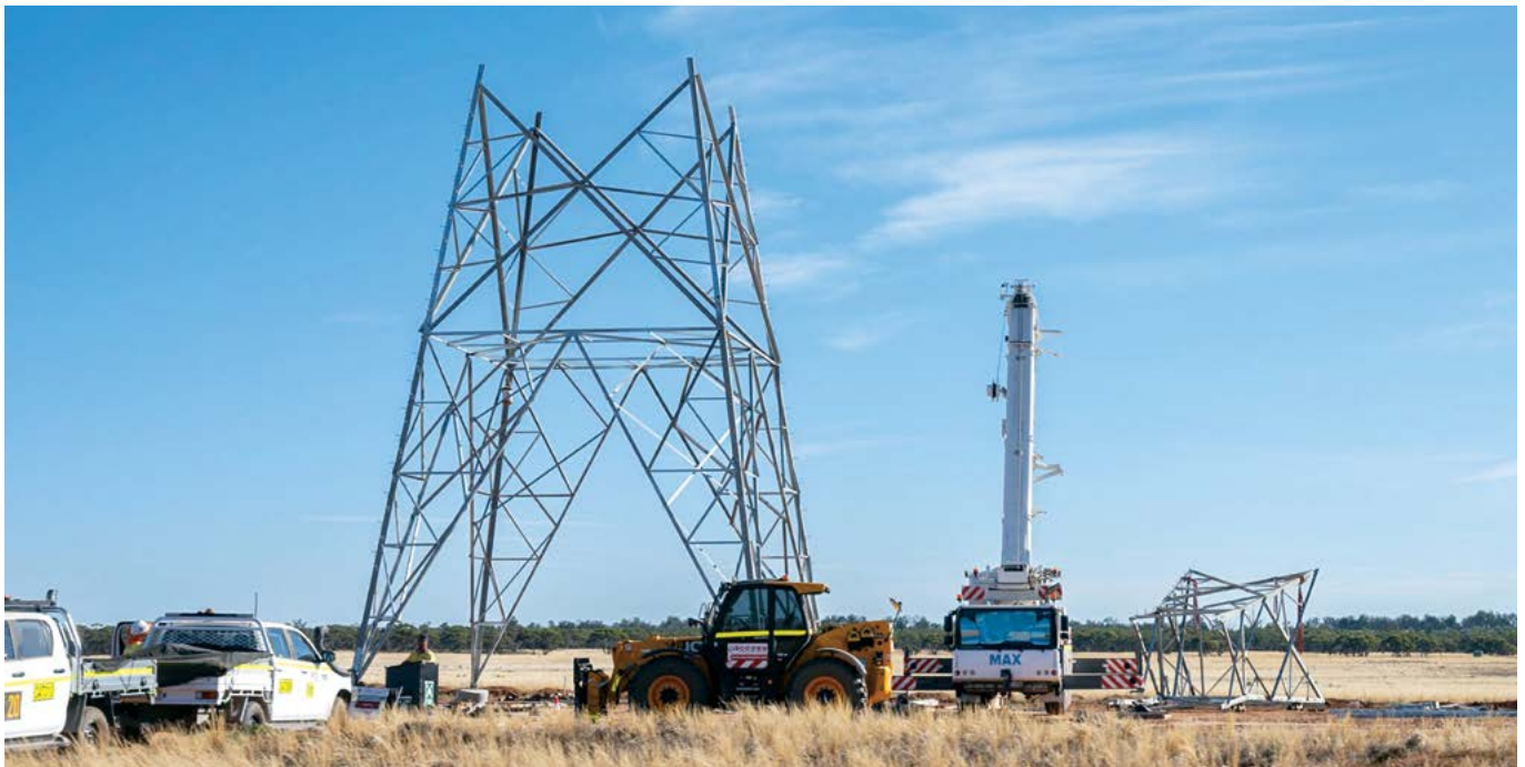
Figure 2: A 500 kV transmission tower being assembled onsite.
