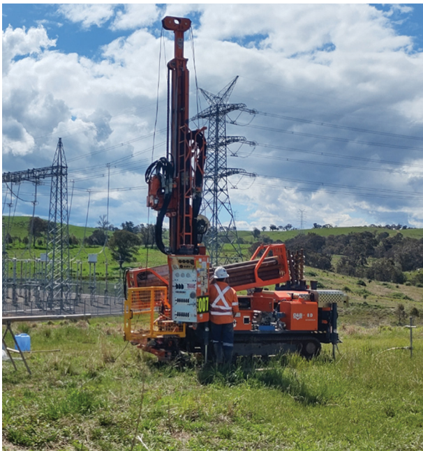
Pictured: Geotechnical investigations at Bannaby substation.
