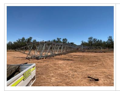
Photo 1: Towers ready for erection
