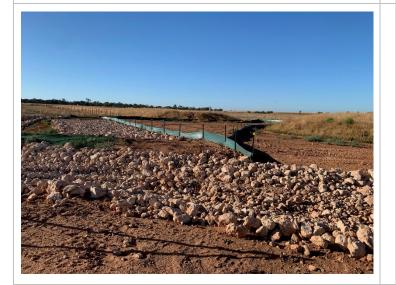
Photo 5: Rock lined channel and sediment fence – Camp 6
