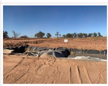
Photo 16: Plastic lined concrete washout pit
