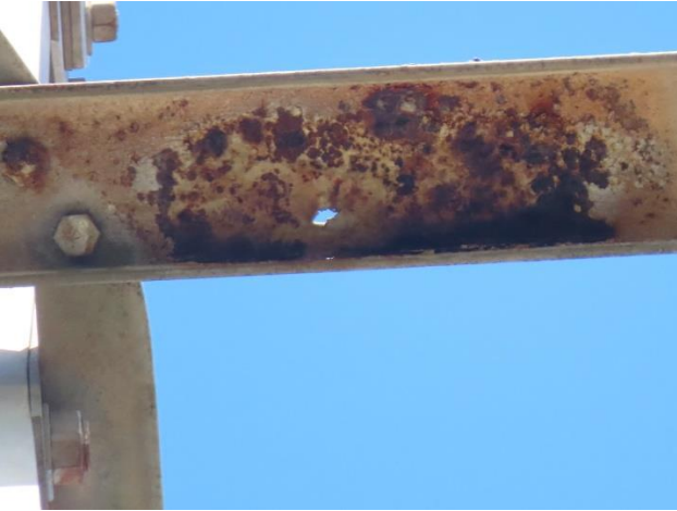
Figure 2-3 Corroded fittings
