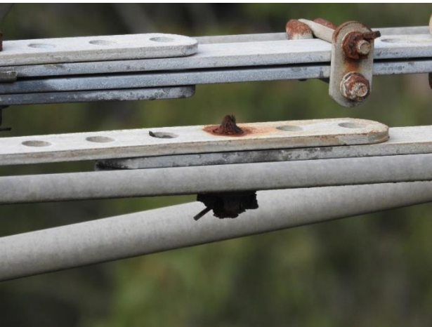
Figure 2-3 Corroded fittings
