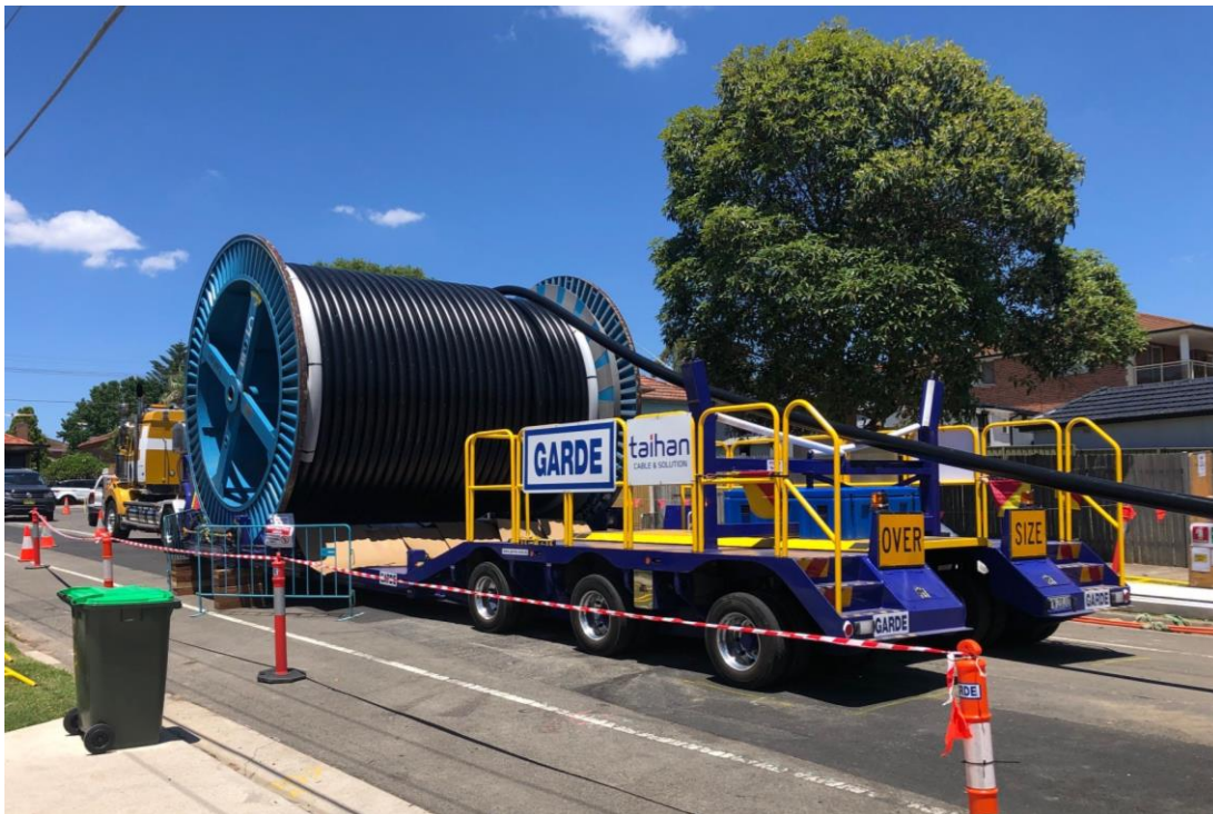
330kV cable installation – Maiden St, Greenacre
