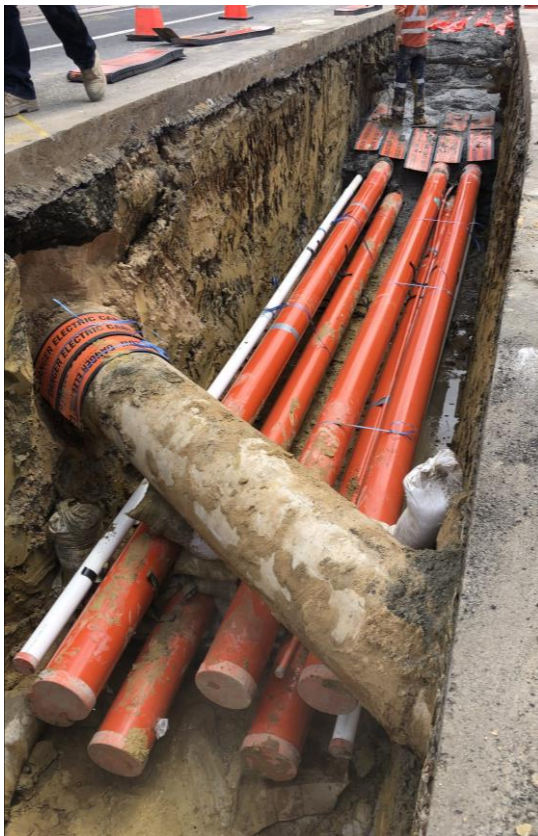
Trefoil arrangement (passing under other service)
