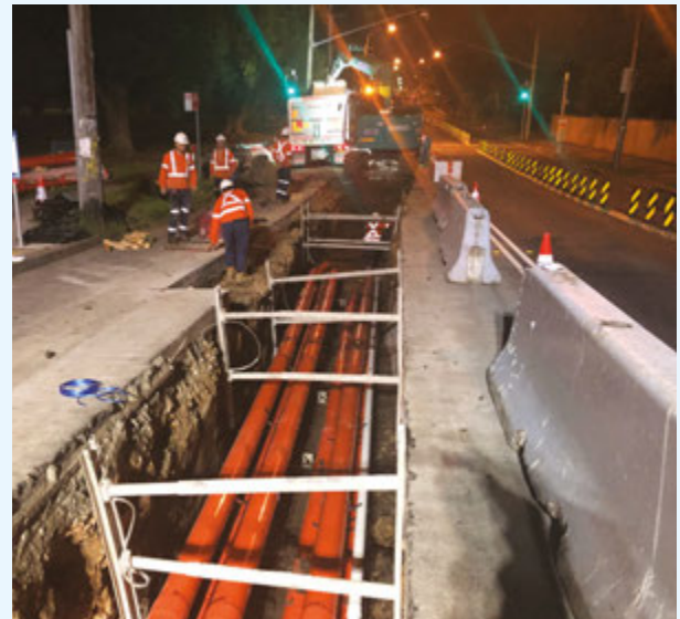
夜間溝槽挖掘施工 (Old Canterbury Road, Ashfield)
