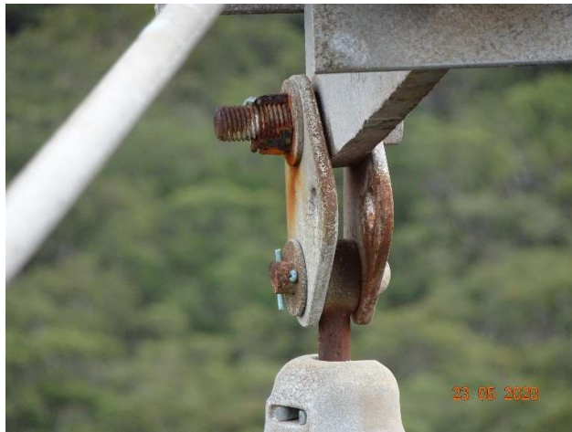
Figure 2-4 Tower earthing issues
