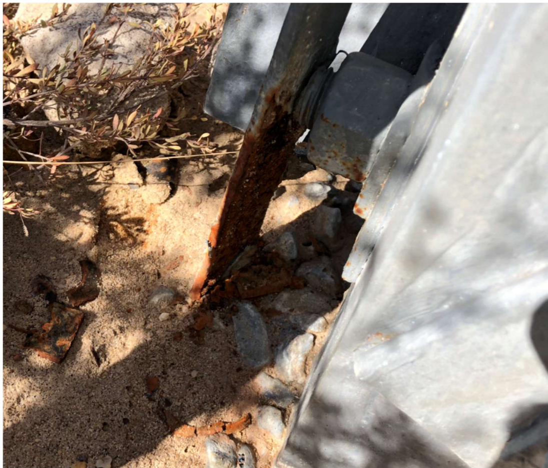
Figure 2-4 Tower earthing issues
