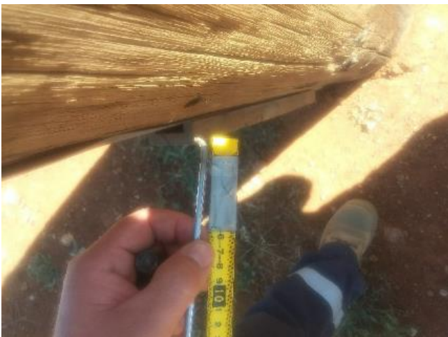
Figure 2-5 Measured hollow section at pole
