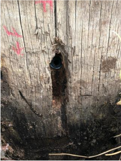
Figure 2-5 Measured hollow section at pole
