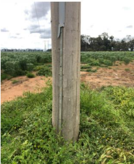
Figure 2-3 Broken Batten
