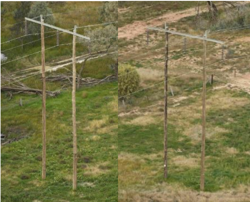
Figure 2-2 shows wood pole structures on Line 94U.
