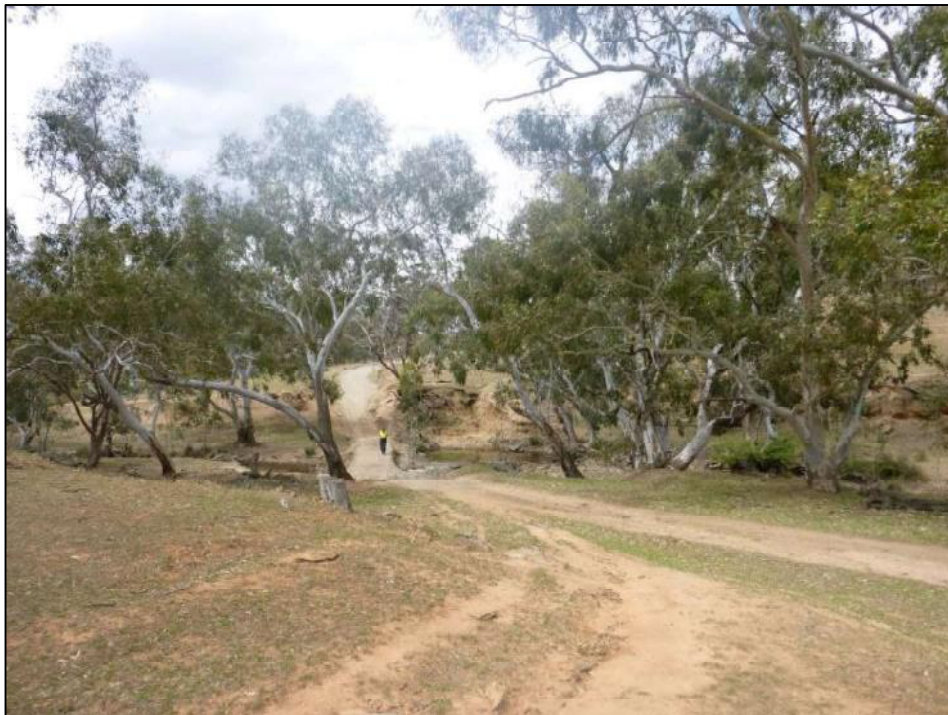
Plate 8: View northeast towards the creek crossing requiring upgrading between Structures 99–100.
