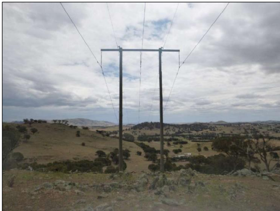
Plate 4: View northwest to Structure 94A.
