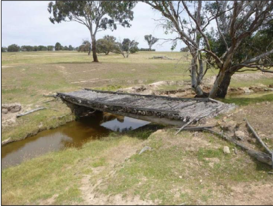
Figure 4-1: View of the old wooden bridge between Structures 89–90.
