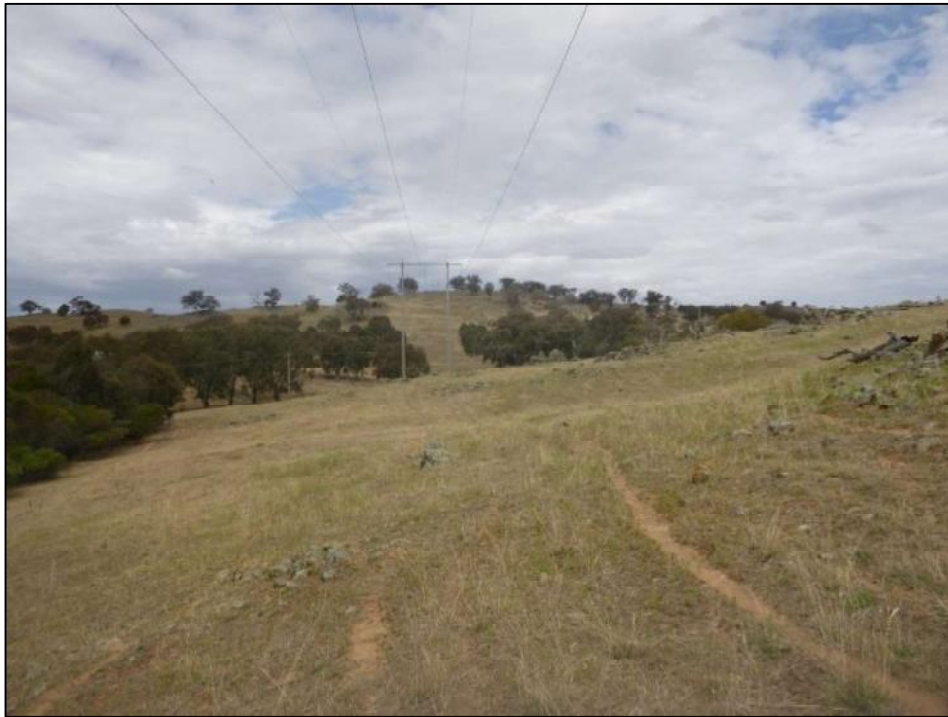
Plate 7: View east towards proposed landscaping area between Structures 95 and 96.
