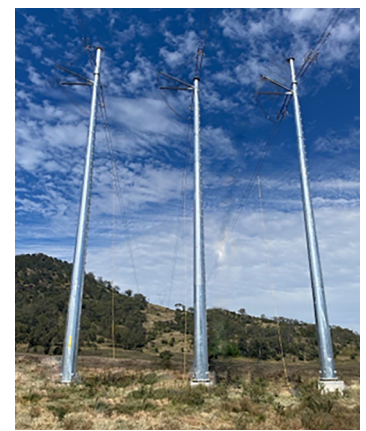
An example of a three pole configuration.
