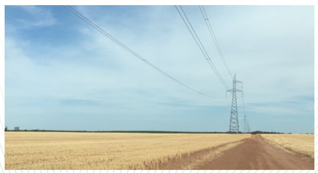
Existing transmission line near Balranald, NSW
