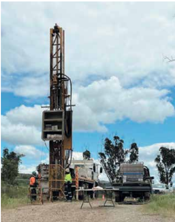
Image: Truck mounted drill rig on site.
