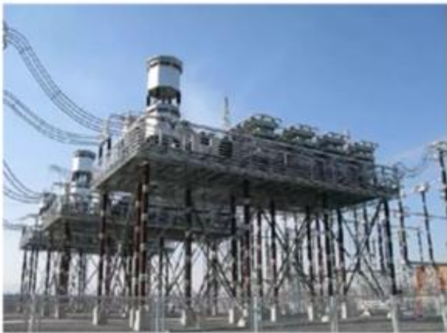
VNI West Power Flow Controllers
