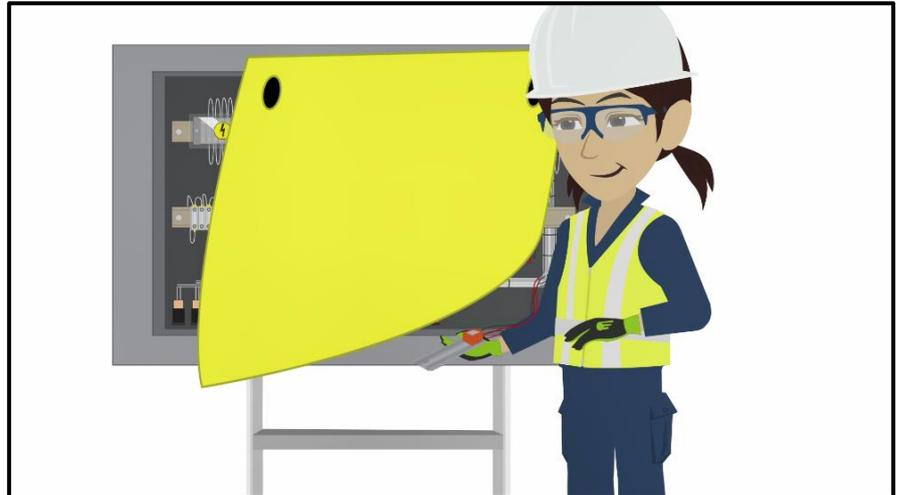
Barriers for work on or near live ELV or LV conductors must have insulation rating appropriate for the work and their condition inspected prior to commencing an activity.
