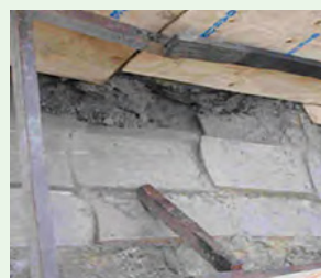
Below ground concrete cable cover slabs
