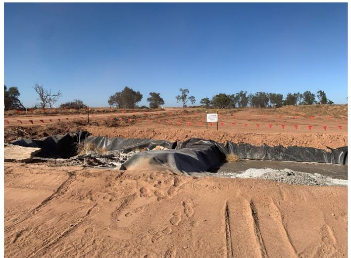
**Photo 16:** Plastic lined concrete washout pit
