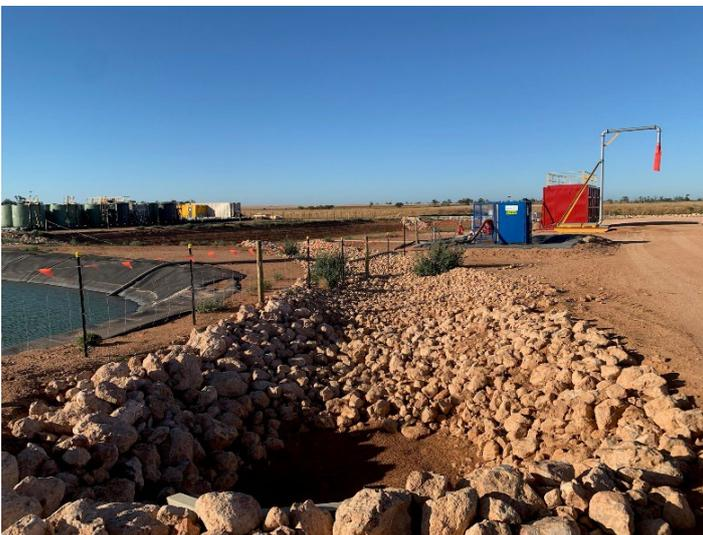
**Photo 9:** Primary basin inlet channel with fire tank and basin dewatering pump in the background
