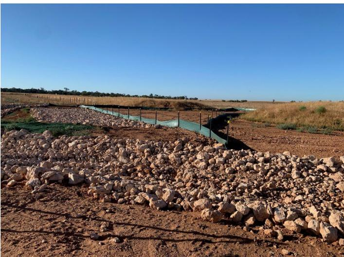
**Photo 5:** Rock lined channel and sediment fence – Camp 6
