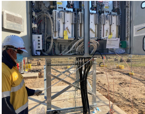
Termination of control cabling
