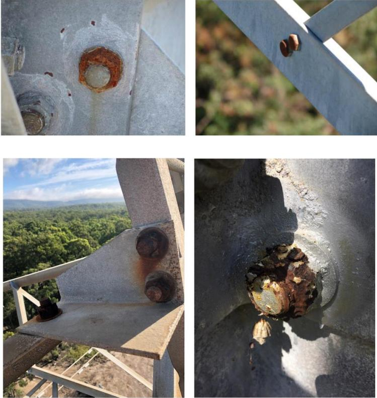
Figure 2-7 Corrosion affecting tower members
