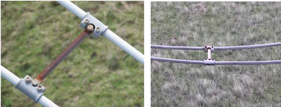
Figure 2-5 Corrosion affecting conductor fitting attachments
