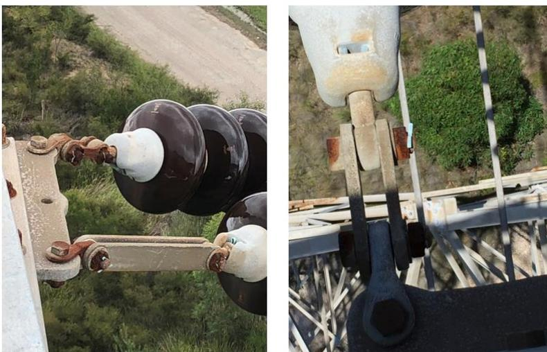
Figure 2-6 Corrosion affecting tower fasteners
