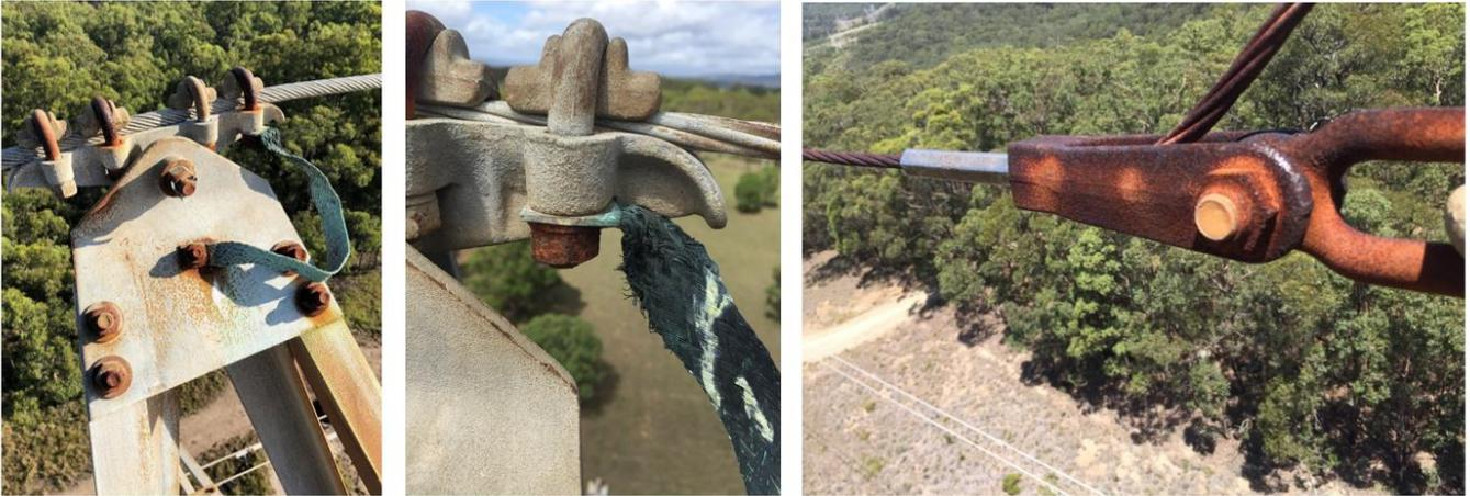
Figure 2-9 Damaged insulators
