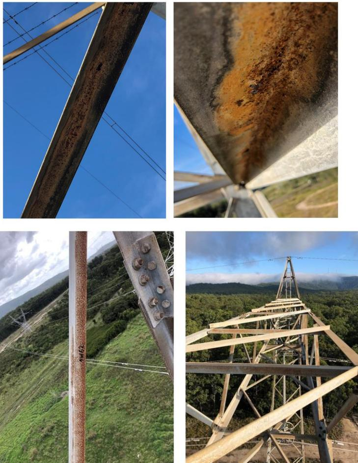
Figure 2-8 Corrosion affecting earthwire fittings
