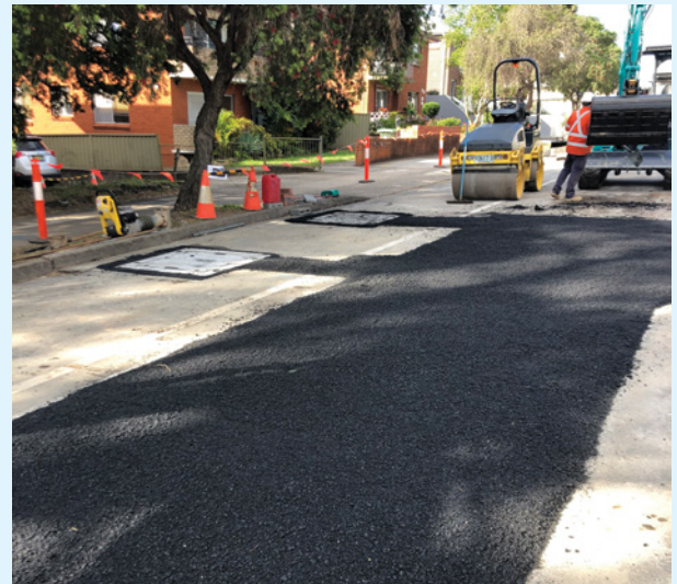
Temporary road restoration, Yangoora Road, Lakemba
