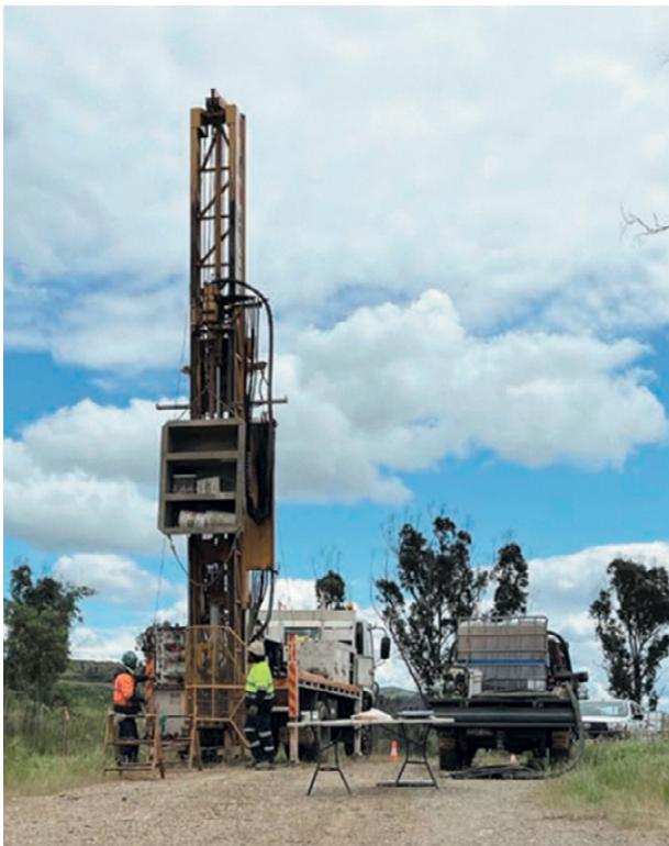
Image: Truck mounted drill rig on site.
