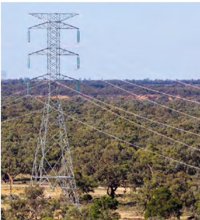
Image: A completed tower on Line 1.
