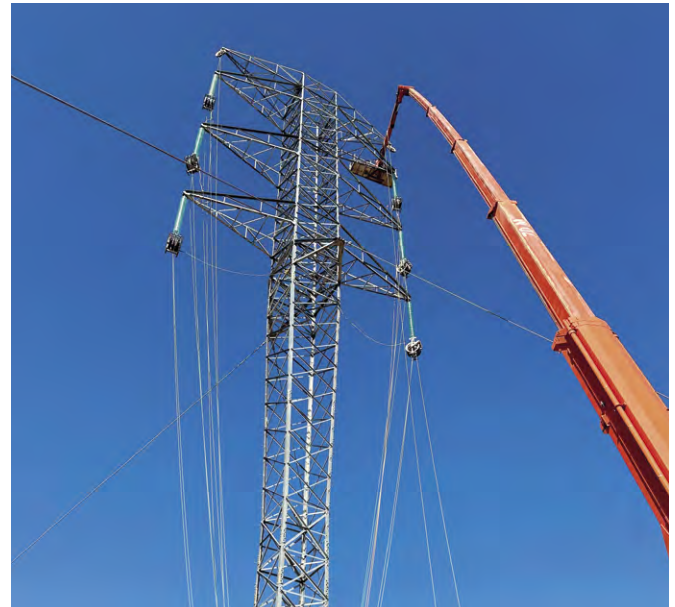
Image: Stringing works on Line 2.
