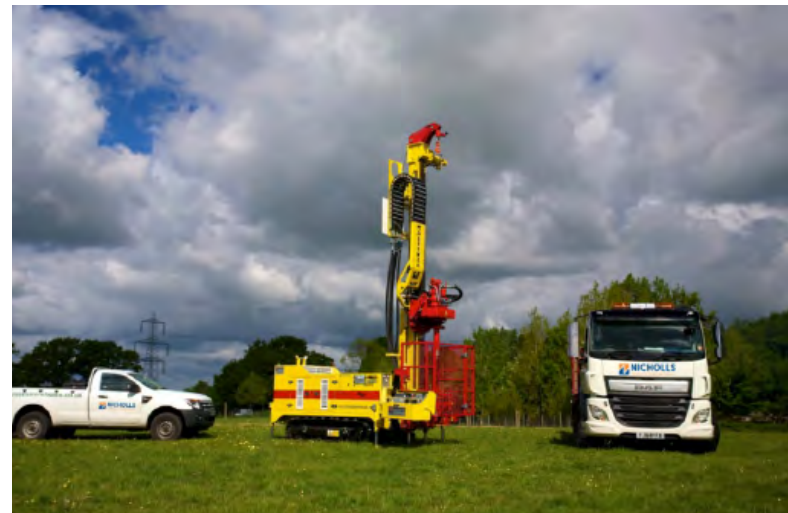
Image: A standard bore rig with drill and support vehicle.
