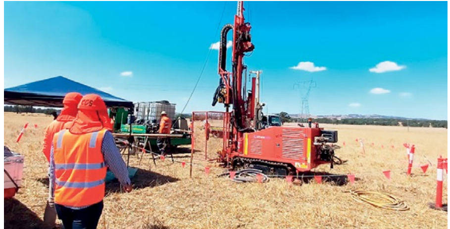
Image: HumeLink West conducting geotechnical investigations.
