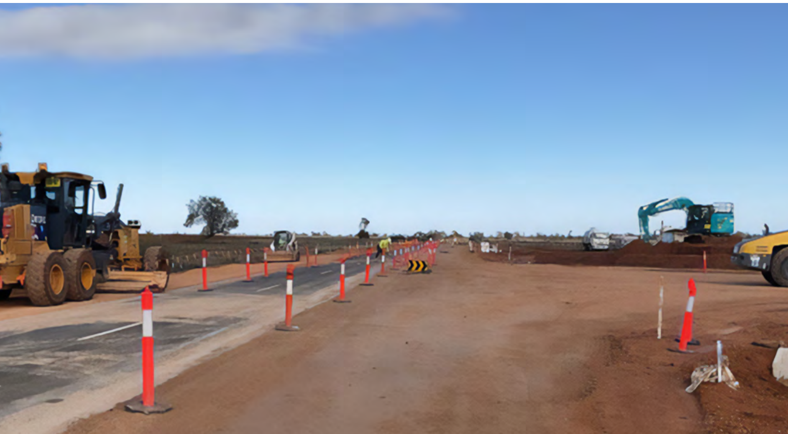
Image: Example of access point works on Transgrid's EnergyConnect project.
