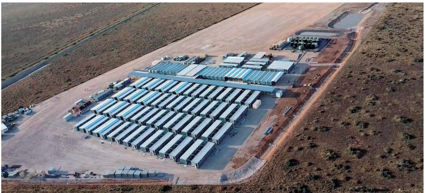
Image: Example of an established temporary worker accommodation camp site (Cobb Highway, Booroorban) currently in use as part of the EnergyConnect (NSW – Eastern section) project
