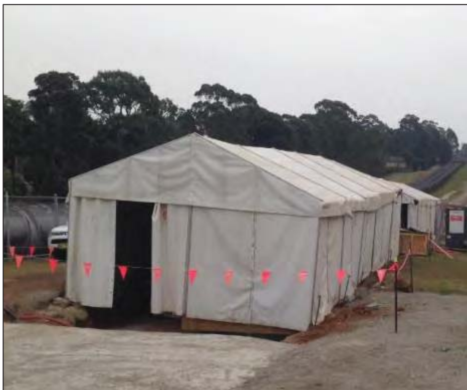
Figure 3-5: Temporary joint bay hut
