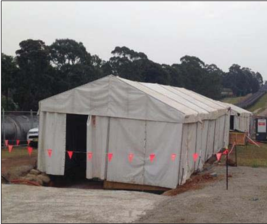
Figure 4-7: Temporary joint bay hut
