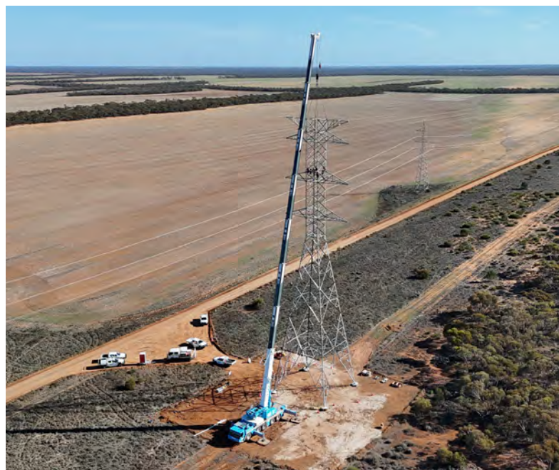
Image: First tower being erected on Line 2 from Buronga to Dinawan.
