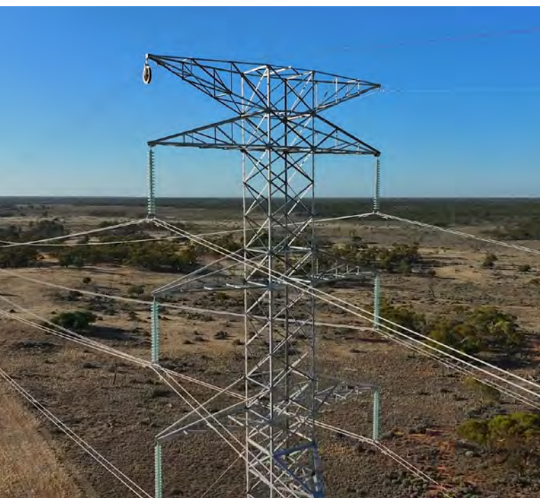
Image: Completed transmission towers on Line 1.
