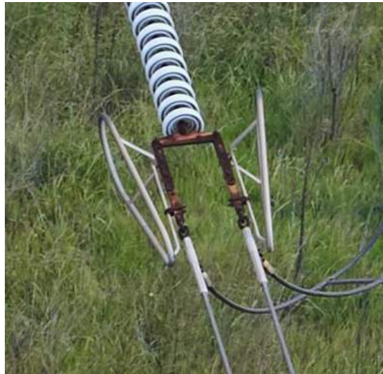
Figure 2-4 Corroded insulator pins
