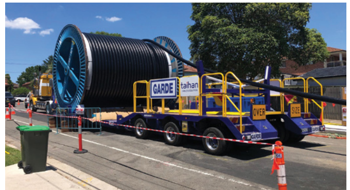
Delivering and pulling cable into the conduits at Maiden Street, Greenacre
