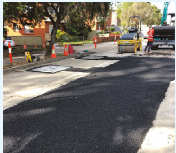
临时道路表面修复 (Yangoora Road, Lakemba)
