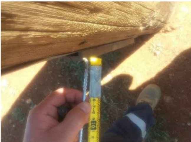
Figure 2-5 Measured hollow section at pole
