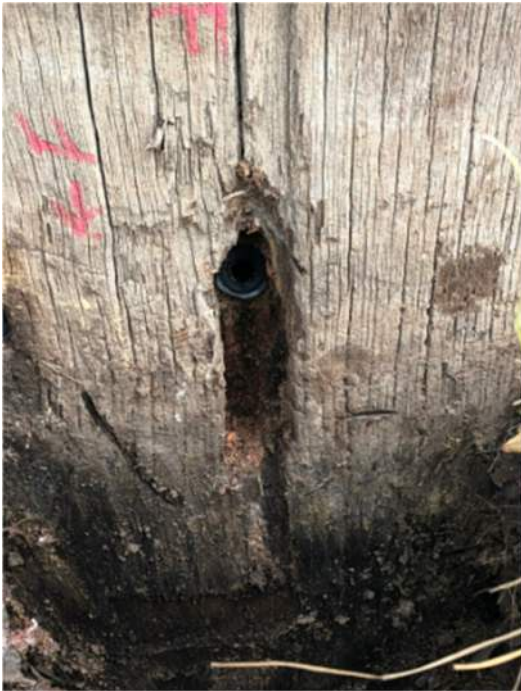
Figure 2-5 Measured hollow section at pole
