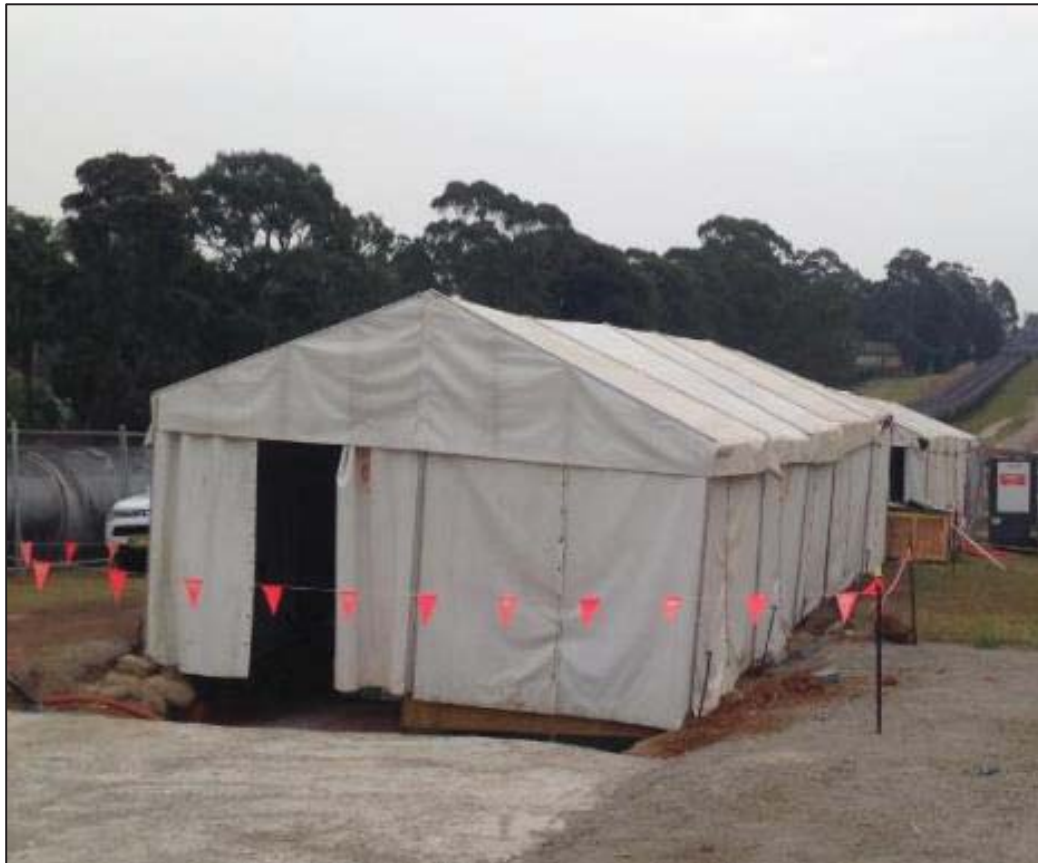
Figure 2-7 Temporary joint bay hut
